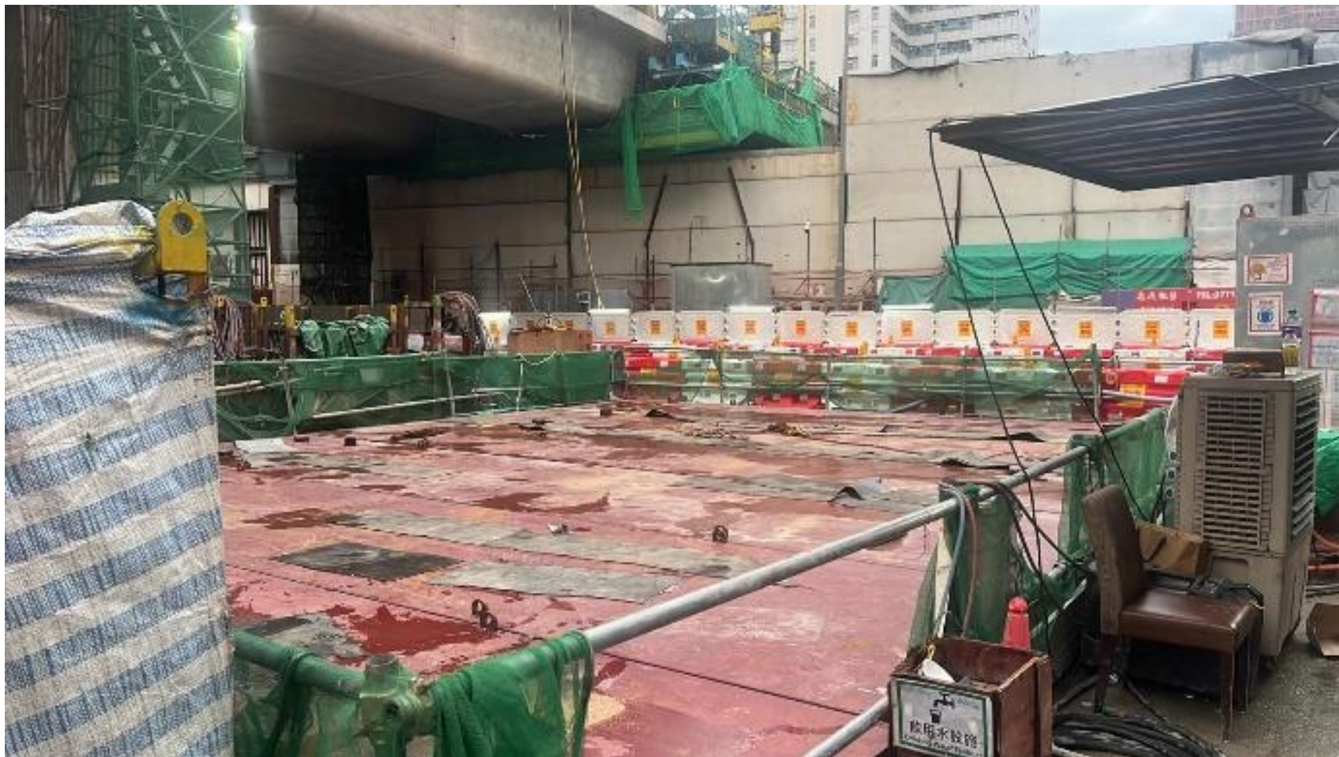
Remark 2: Noise enclosure at Underground Working Zone
